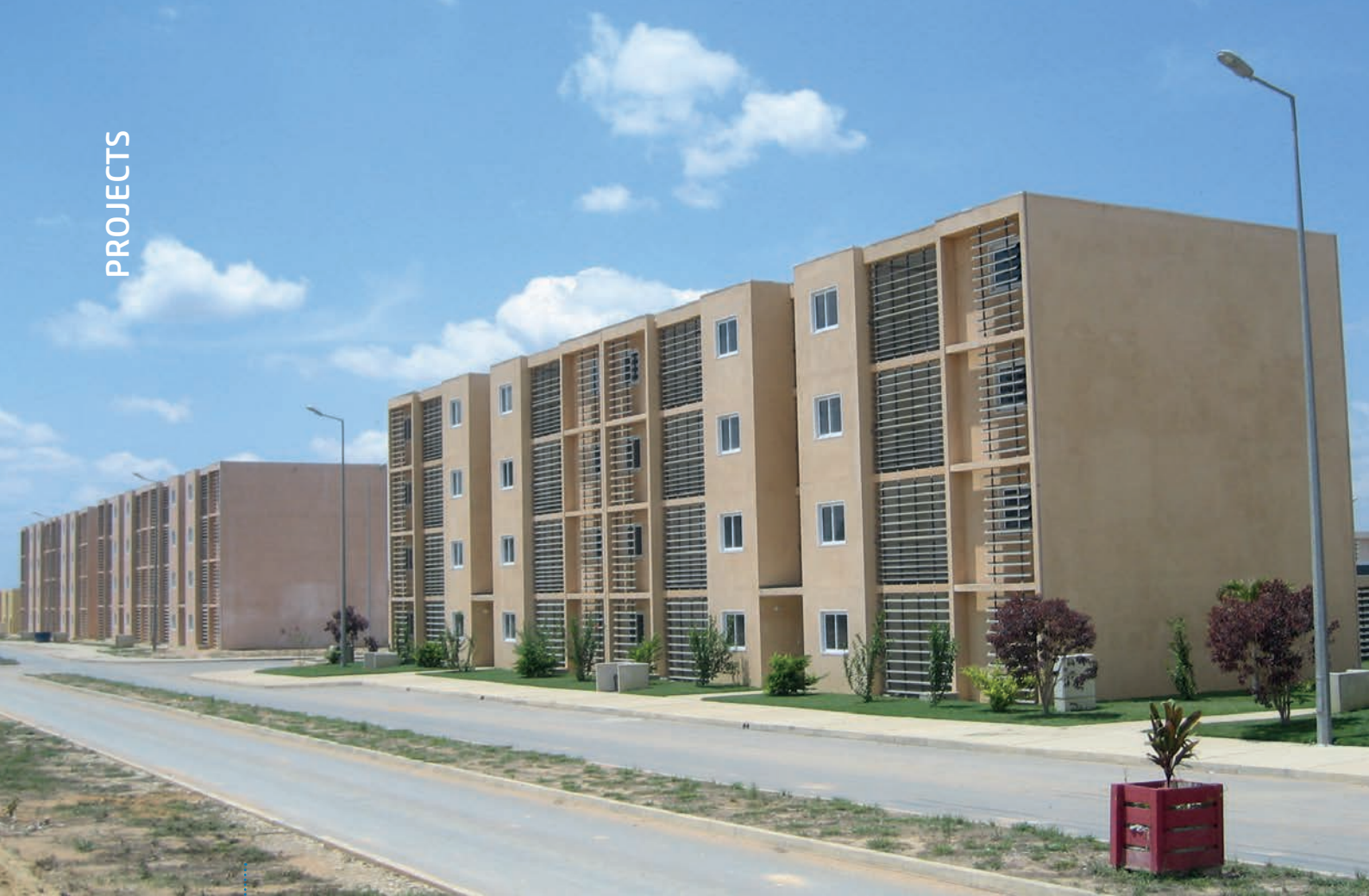
Example of a building unit made of Ytong-AAC
