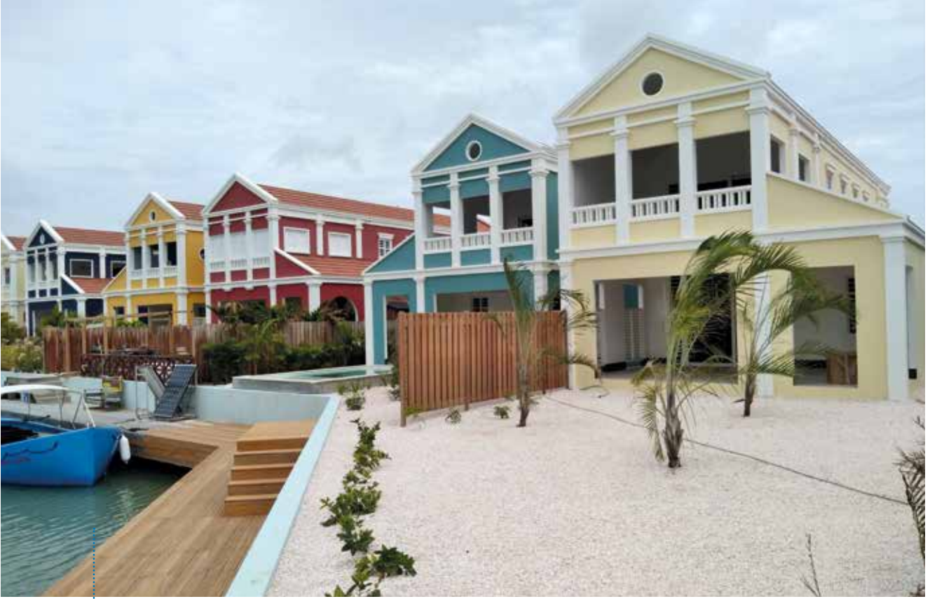
The water villas are located directly on the shoreline and are characterized by a colonial architecture.
